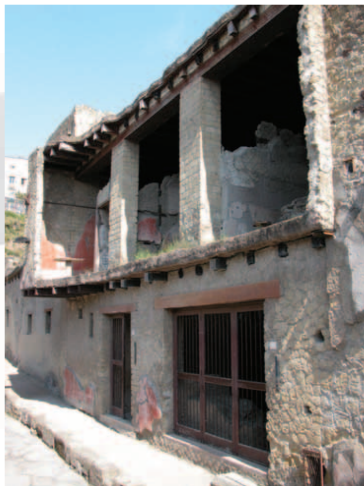
Above: View of the façade, showing the upper floor and balcony.
