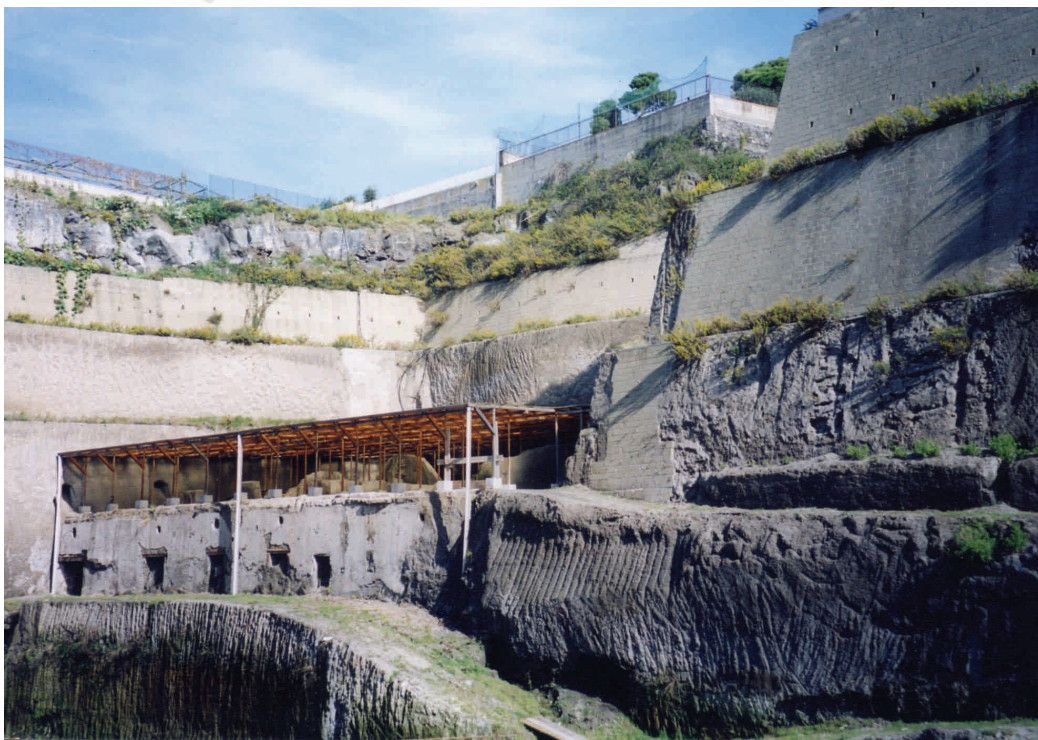
Left: the excavated corner of the Villa, covered by a fibreglass roof, with the volcanic rock that encases it looming overhead.
