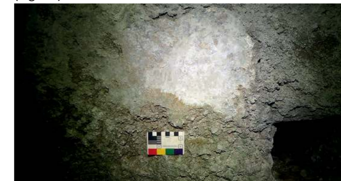
Fig. 5A. A portion of surviving bright white waterproof lining on the wall of the pool of the caldarium .
