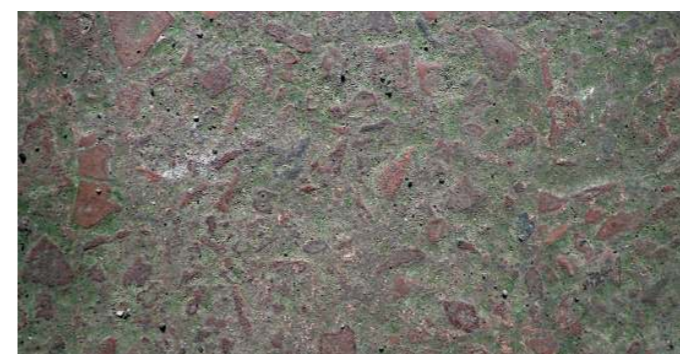
Fig. 4A. The cocciopesto floor of the cruciform natatio with roughly reduced terracotta aggregate.
