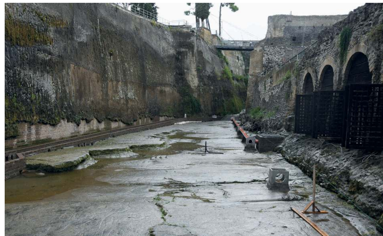
The recently excavated ancient shoreline of Herculaneum with the fornici (so-called boathouses on the right). Once fully excavated the area will be covered in volcanic sand thus recreating the ancient beach.
