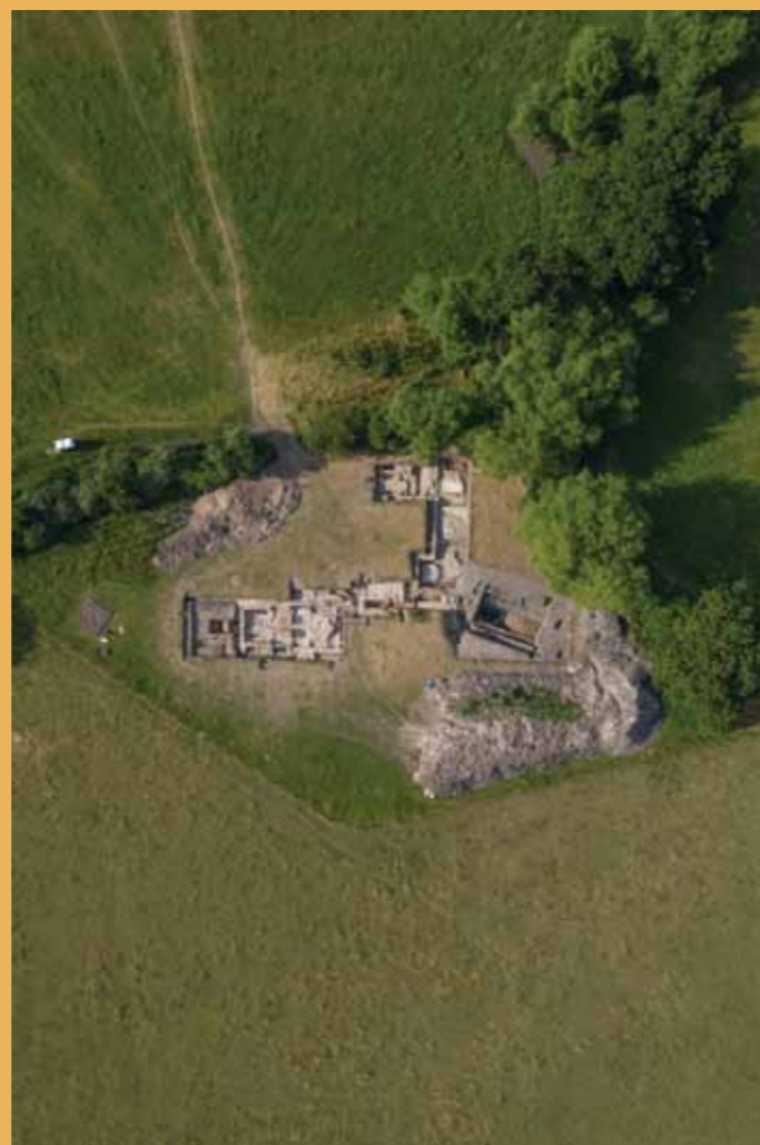
Drone view looking north
